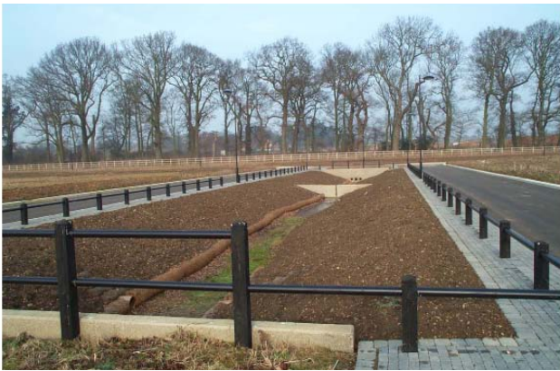
Figure 15.13: Swales at Upton, Northhampton, UK
