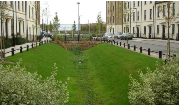
Figure 15.12: Swales at Upton, Northhampton, UK
