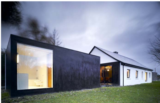
Figure 16.50 : Extension to side of house. Glengowla, Co. Galway. Boyer Kennihan Architects.
