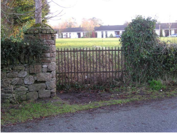
Figure 16.43: Stone wall, pillars and gate, Naas
