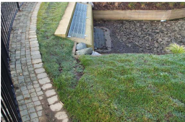
Figure 15.14: Swales at Upton, Northhampton, UK
