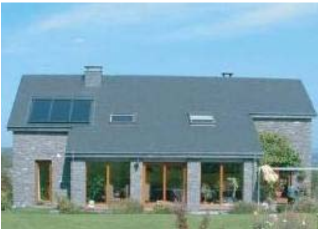
Figure 16.47: Image of roof solar panel
