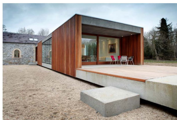
Figure 16.48: Refurbishment and Extension. Ballymahon House. ODOS Architects.
