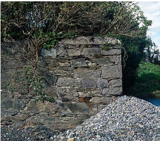
Figure 16.41: Image of traditional stone wall at Devoy Barracks, Co. Kildare
